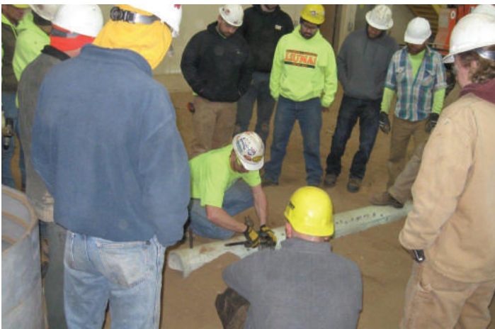
Pipe Class- Tapping Blue Brute C900 Water Pipe
