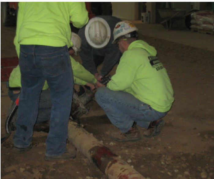
Pipe Class- Tapping Ductile Iron Water Pipe
